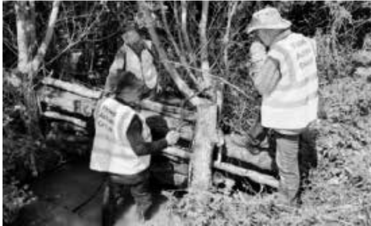
One of the dams where the height has been raised and secured with ratchet lashings. Left to right, Mike McCarthy, John Dinnie and Trevor Bradnam.
